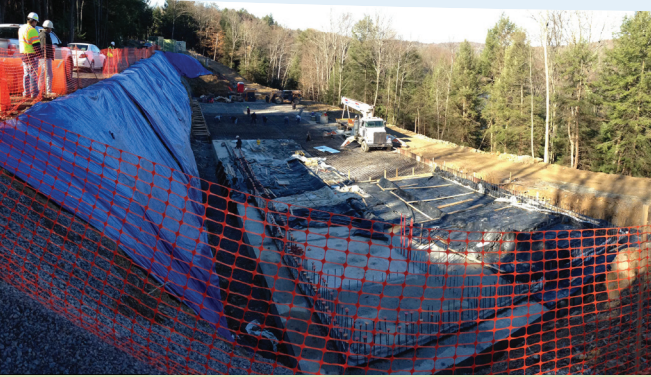
Construction underway on the foundation of the new Liberty lift station.
